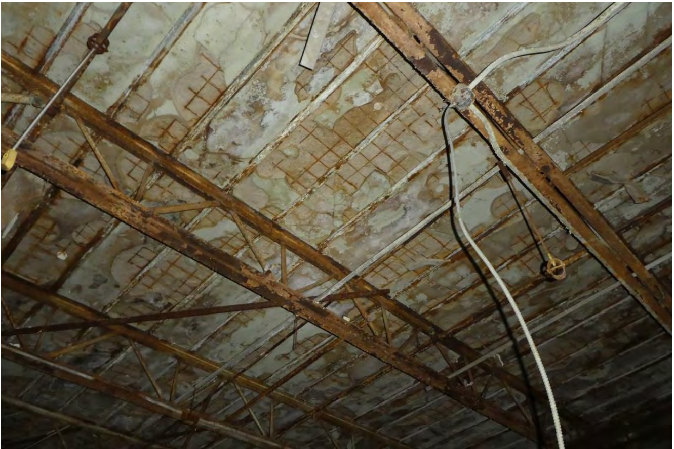
Photo 20: Building 21 roof, looking northwest.
