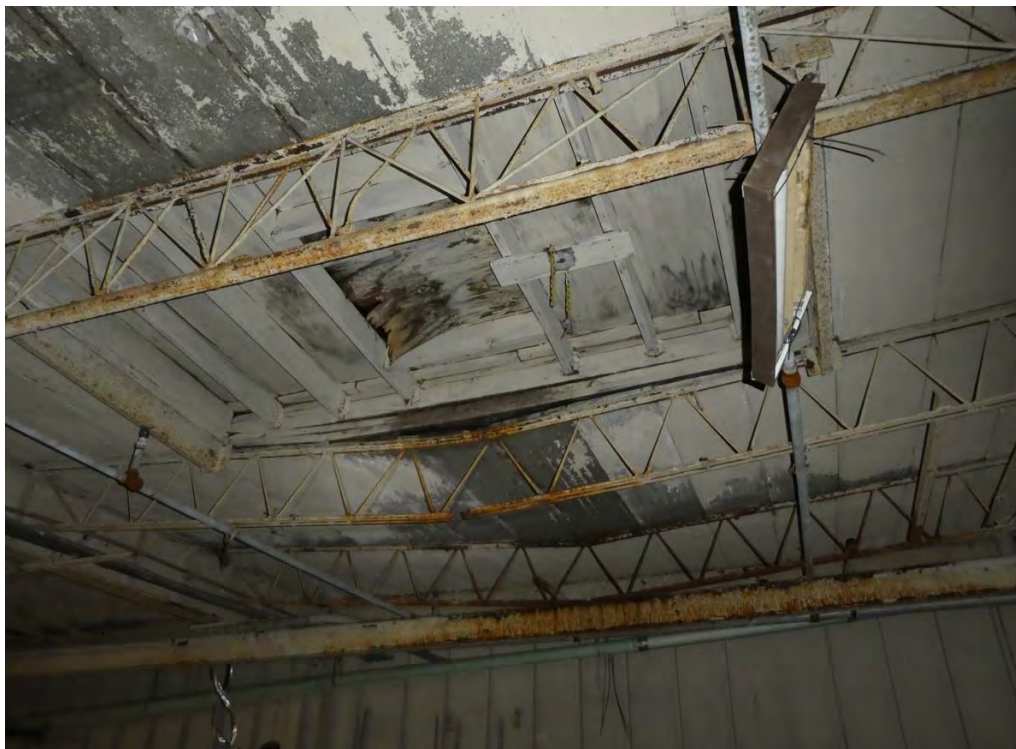
Photo 19: Building 20 presumed skylight infill, looking west.
