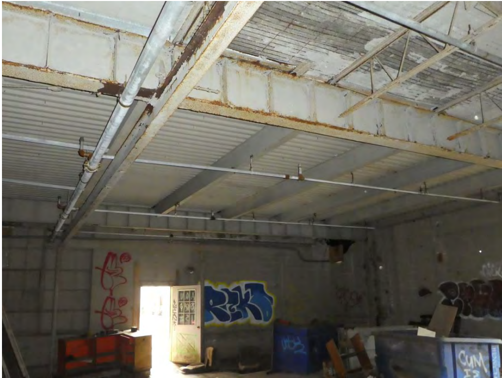
Photo 18: Building 20 roof deck transition, looking northeast.
