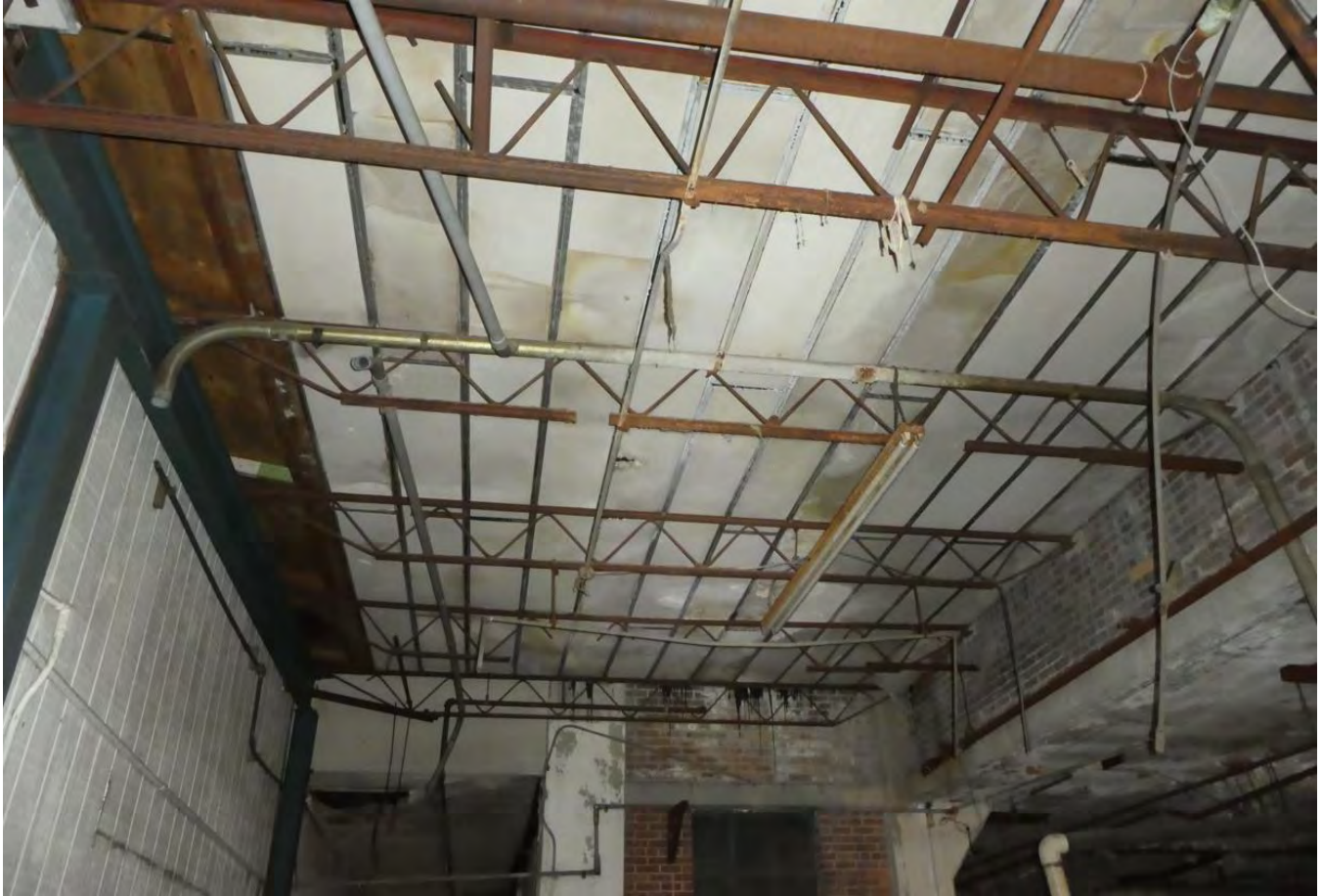
Photo 21: Building 22 roof, looking west.
