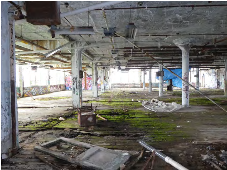
Photo 1: Building 1, Third Floor
