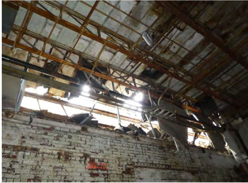
Photo 3: Building 3, looking south at Building 5 roof.
