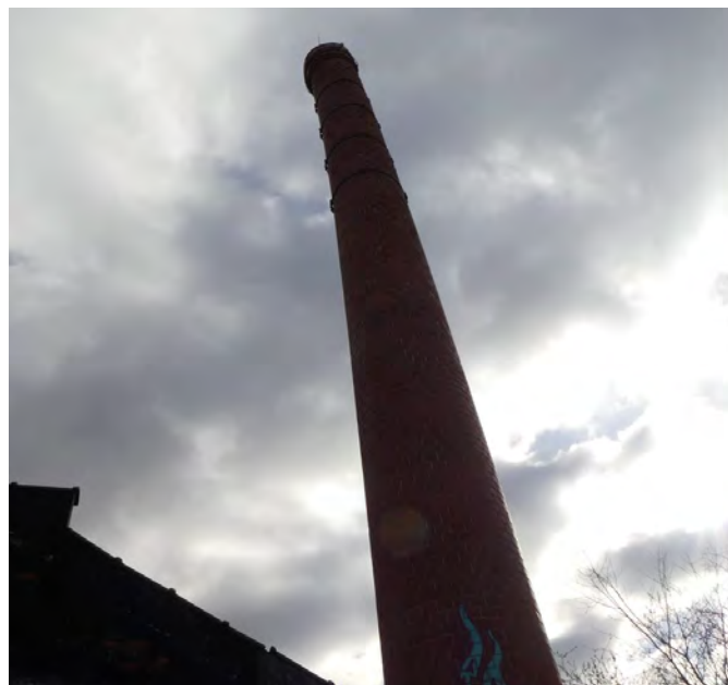
Photos 63 and 64: 74-foot-tall Boiler stack
