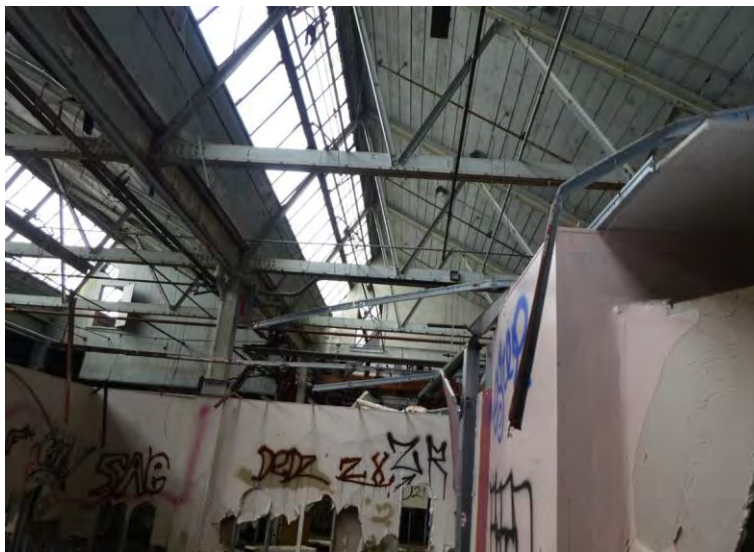
Photo 4: Building 4, looking east up at sawtooth roof.
