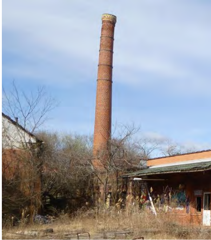
Photo 22: 75-foot-tall Boiler Flue Stack.
