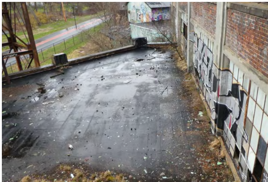
Photo 13: Building 16, roof, looking north.
