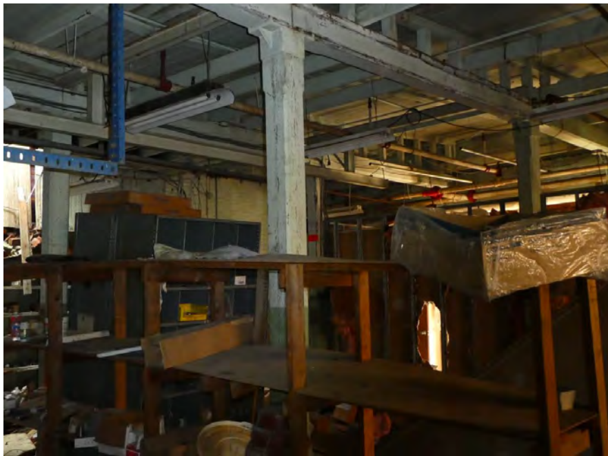
Photo 7: Building 7, looking southeast.
