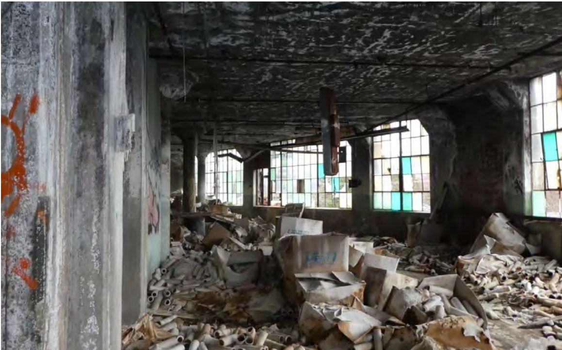
Photo 14: Building 17, third floor, looking west.
