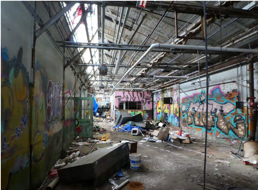
Photo 5: Building 5, looking east up at sawtooth roof.
