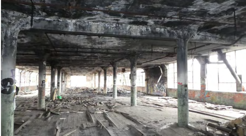
Photo 9: Building 10, third floor, looking east.
