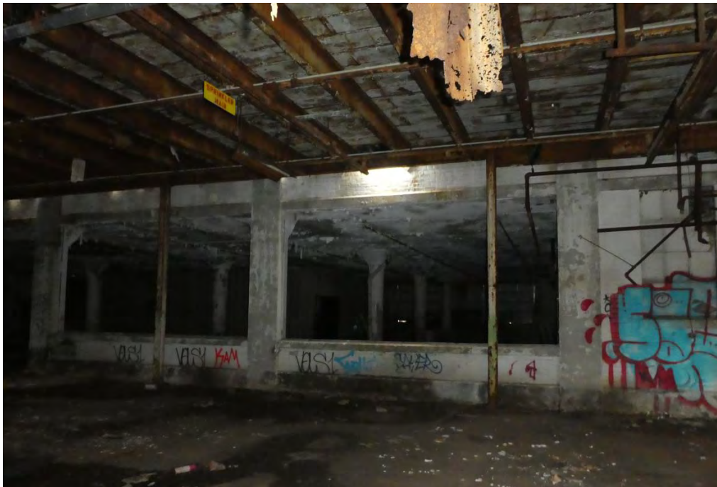
Photo 2: Building 2, looking north at Building 1 first floor.
