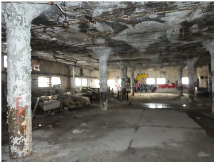
Photo 10: Building 11, first floor, looking east.
