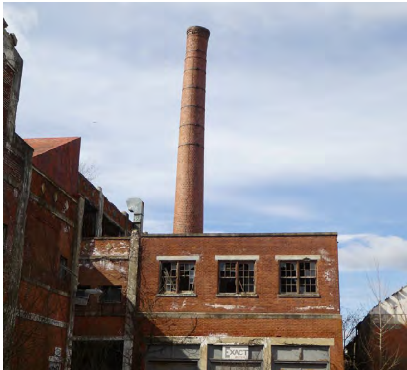
Photo 23: 98-foot-tall Boiler Flue Stack.
