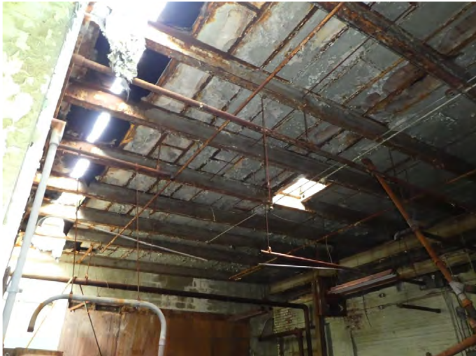
Photo 8: Building 8, looking southeast.
