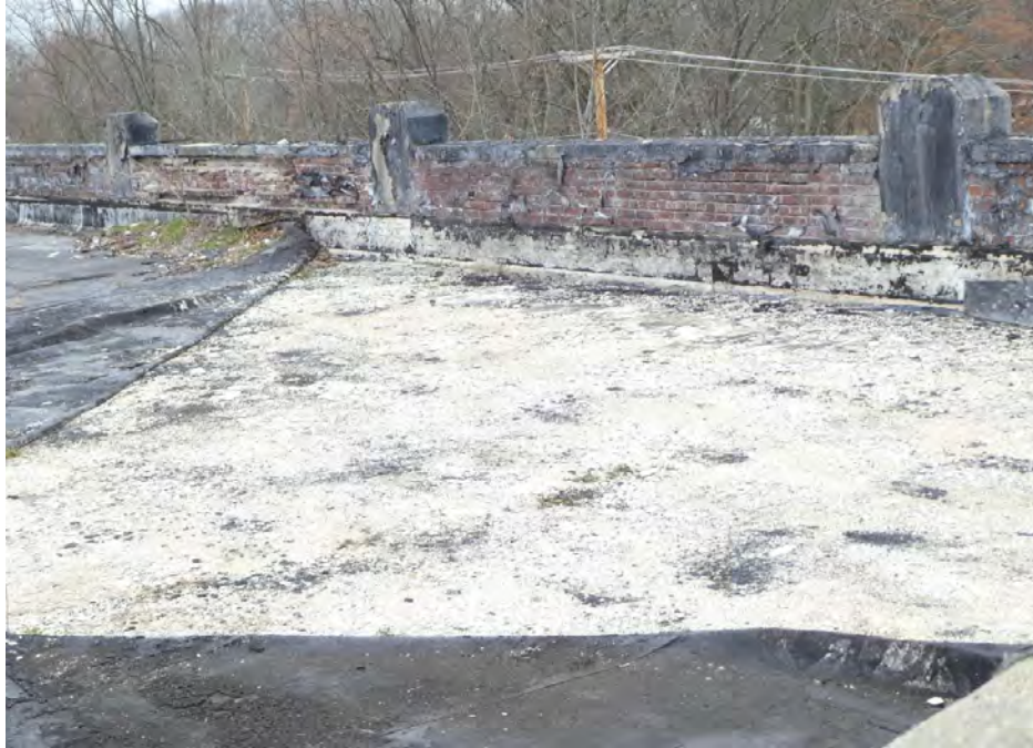
Photo 30: Building 14, existing membrane roof pulled from roof deck and parapet.
