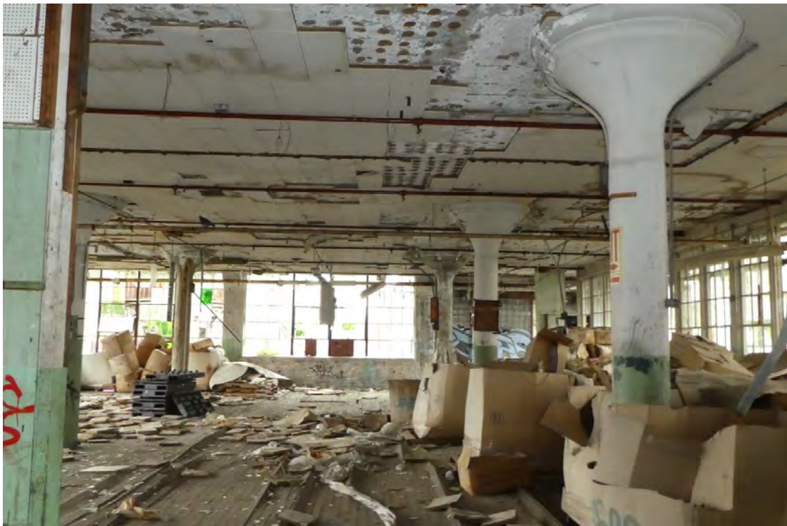
Photo 11: Building 12, third floor, looking north.
