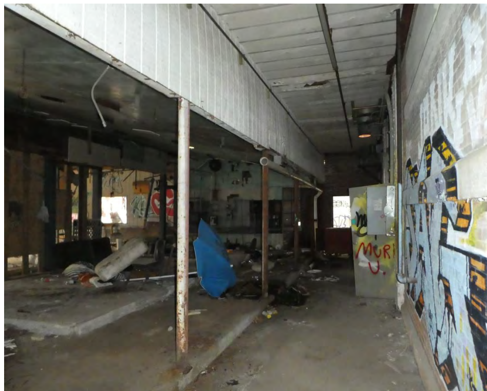
Photo 15: Building 18, ground floor, looking west.
