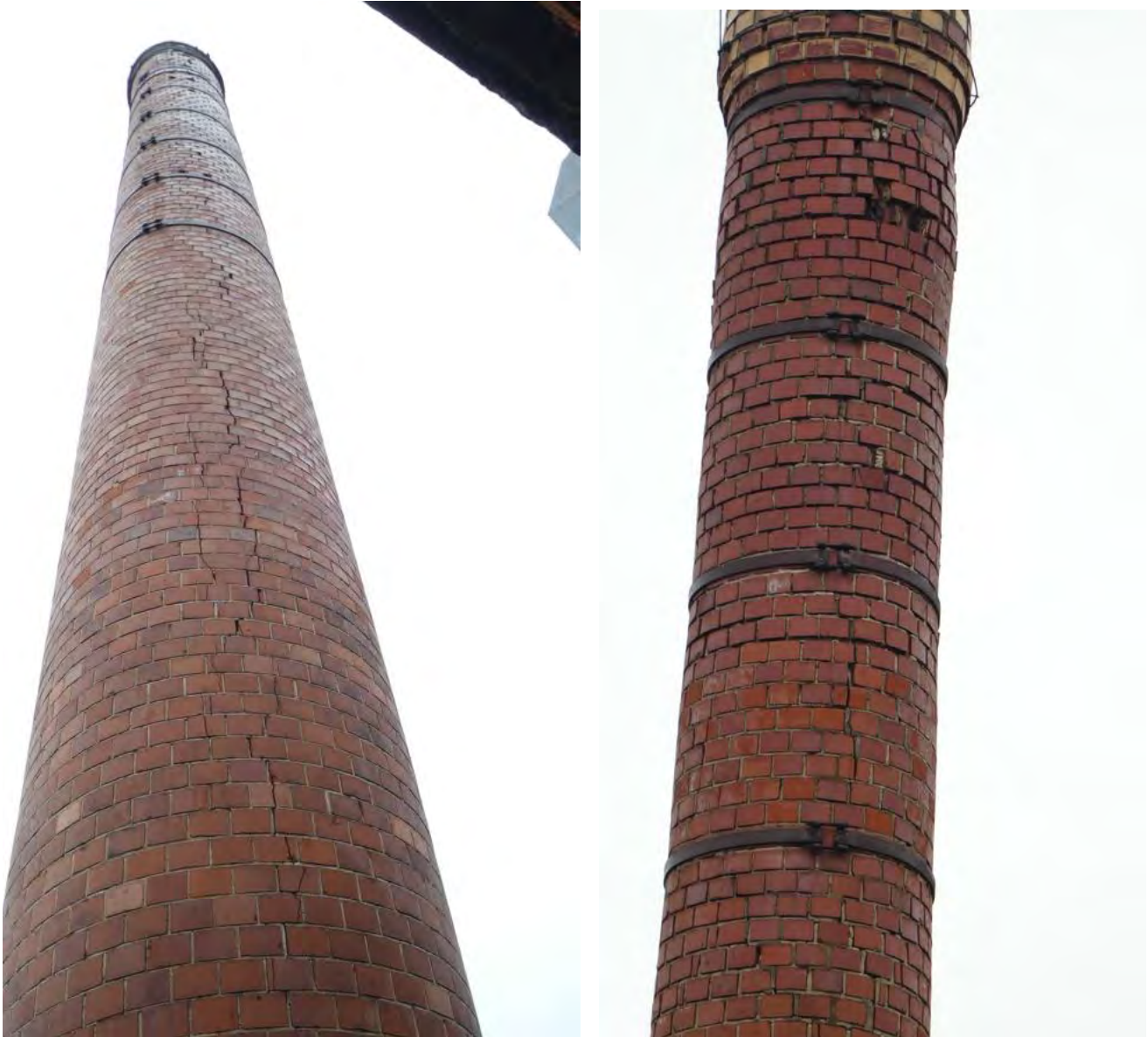
Photos 65 and 66: 98-foot-tall Boiler stack
