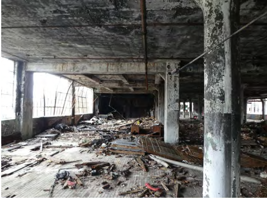
Photo 12: Building 13/14, second floor, looking north.
