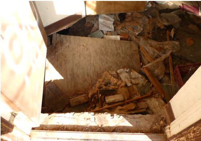
Photos 53 and 54: Building 7, images of floor collapse.
