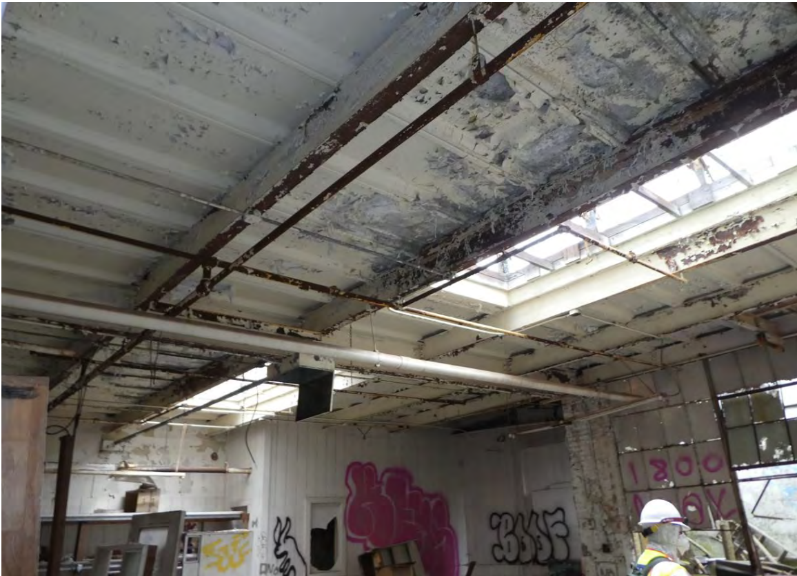
Photo 17: Building 19 roof and skylights, looking northeast.
